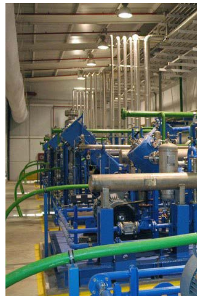
Figure 4b: Compressor station
